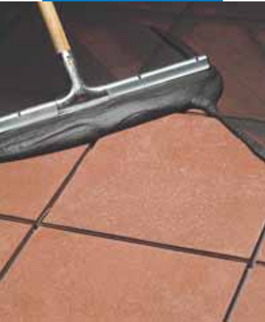
Grouting a terracotta tile floor with float
