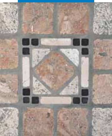
An example of a grouted antique marble stone floor
