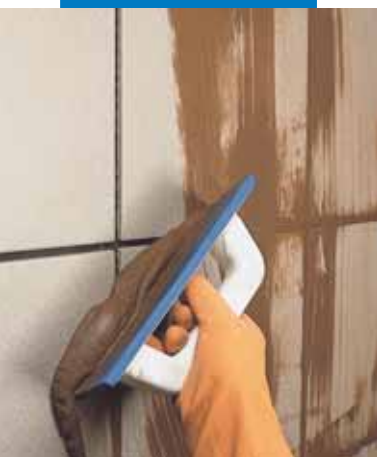
Grouting an external wall with a float
