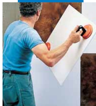
Laying KERAION on a wall
