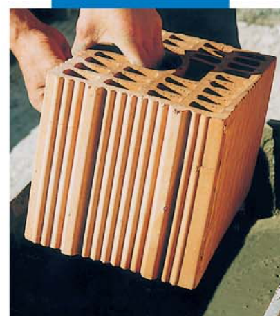
Dipping a concrete block in Adesilex P4
