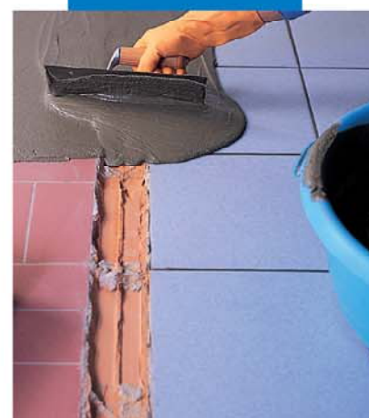
Smoothing existing flooring with Adesilex P4
