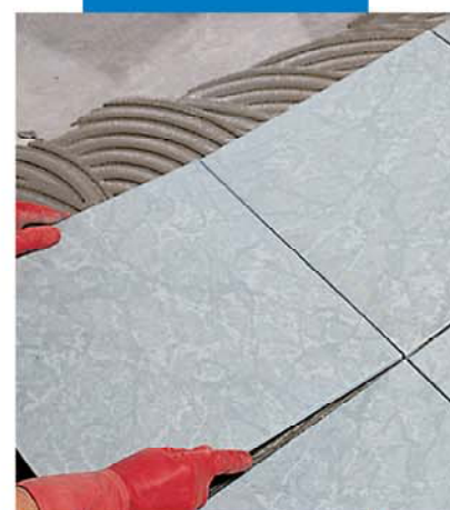
Laying porcelain tiles
