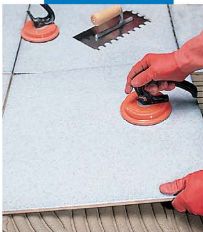
Laying large size tiles
