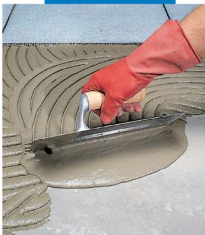
Spreading with semicircular notched trowel
